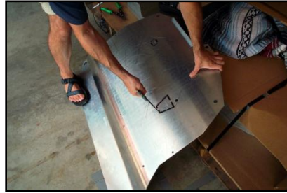
Figure 61 - Cutting the two connecting webs of aluminum
