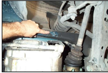
Figure 54 - Pushing their star nuts onto the threaded stud on the bottom side of the frame rail
